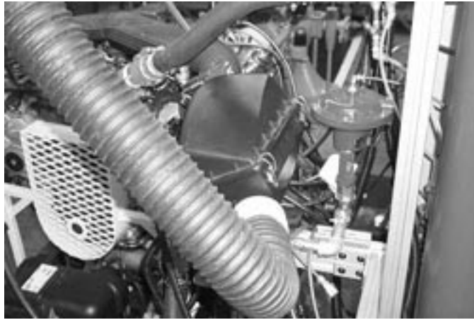
FIG. A3.21 Intake Air Supply System, Air Cleaner, Resonator and Idle Load Control
