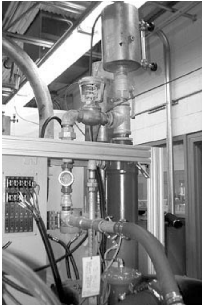
FIG. A3.23 Typical Cooling System, Flow Control Valve, Venturi Flowmeter, Reservoir and Sight Glass
