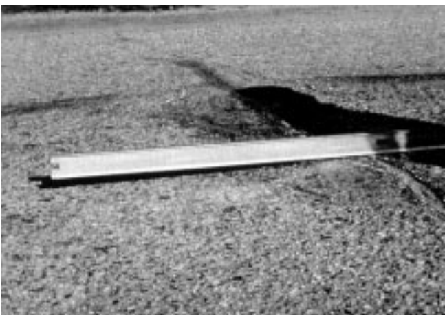
FIG. X1.10 Low-Severity Bumps and Sags
