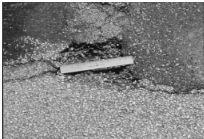
FIG. X1.35 Low-Severity Pothole
