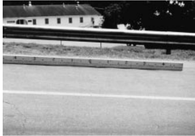
FIG. X1.13 Low-Severity Corrugation
