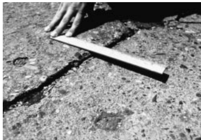
FIG. X2.14 Medium-Severity Faulting
