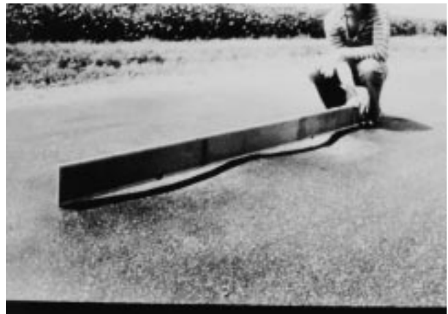
FIG. X1.15 High-Severity Corrugation
