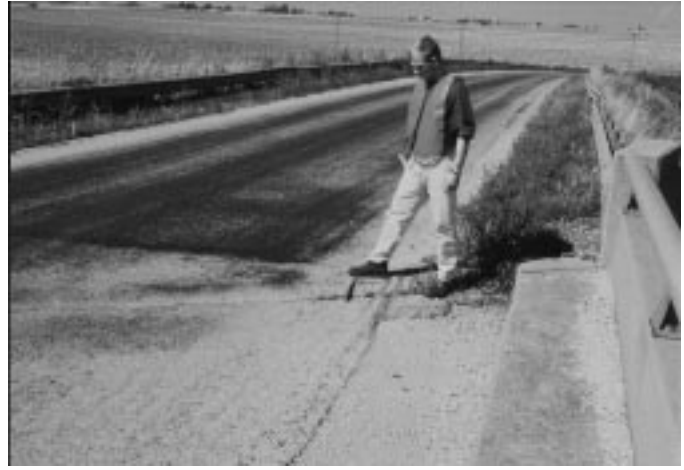
FIG. X1.44 Low-Severity Shoving
