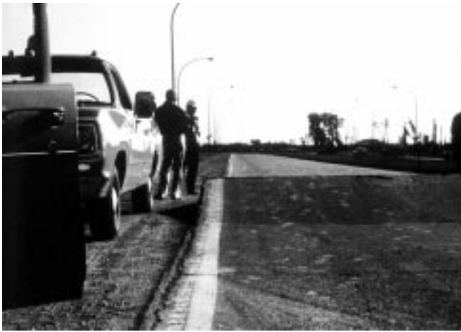
FIG. X2.3 High-Severity Blowup/Buckling
