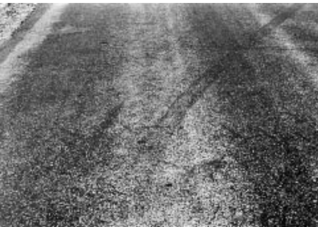
FIG. X1.4 Low-Severity Bleeding
