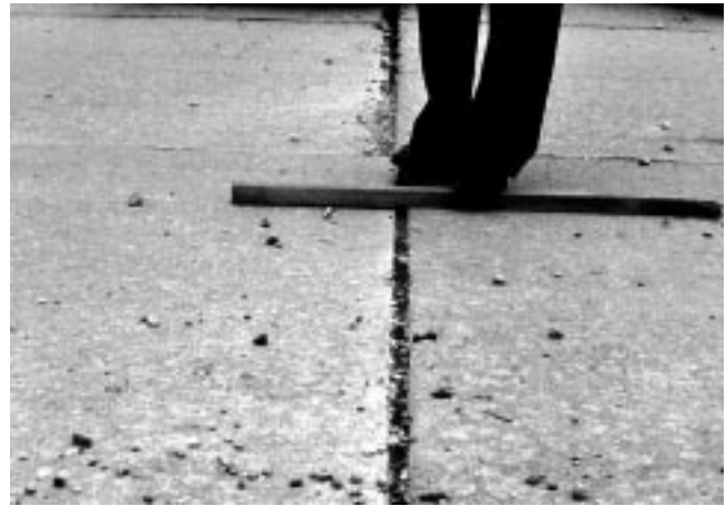
FIG. X2.13 Low-Severity Faulting
