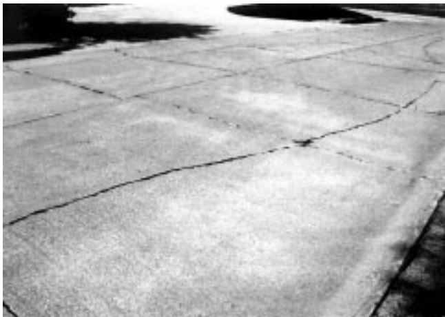
FIG. X2.7 Low-Severity Divided Slab
