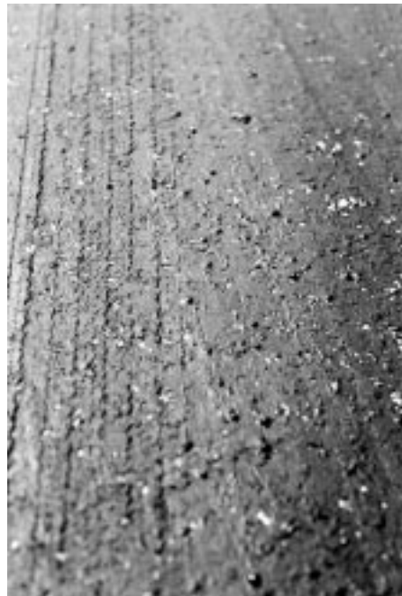
FIG. X1.6 High-Severity Bleeding
