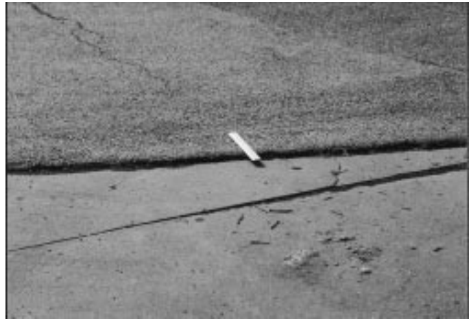
FIG. X1.45 Medium-Severity Shoving
