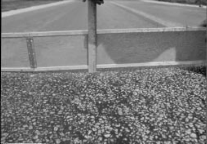
FIG. X1.42 Medium-Severity Rutting
