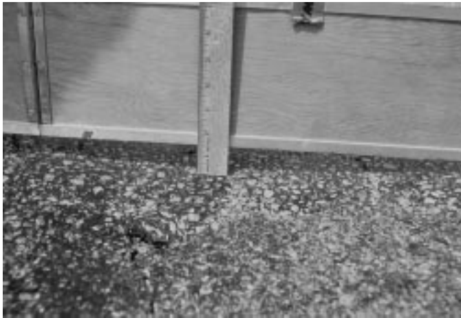
FIG. X1.43 High-Severity Rutting
