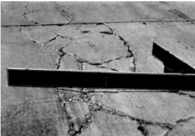
FIG. X2.37 High-Severity Punchout
