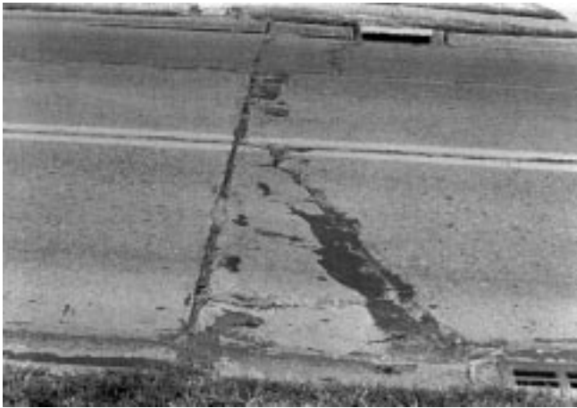
FIG. X2.36 Medium-Severity Punchout
