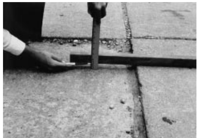
FIG. X2.15 High-Severity Faulting
