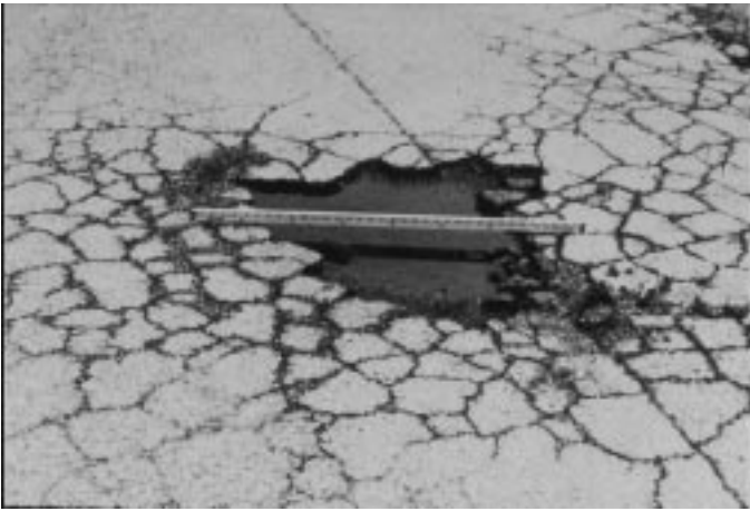
FIG. X1.37 High-Severity Pothole
