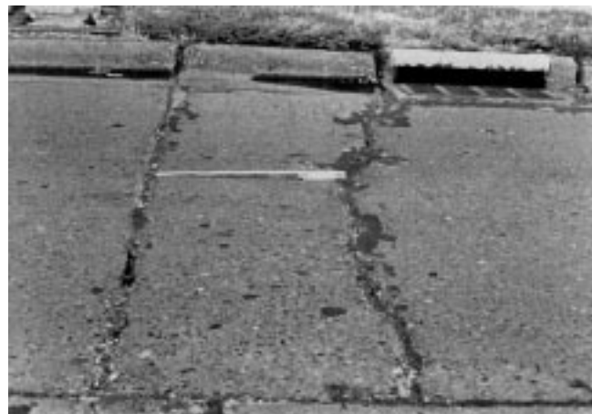
FIG. X2.35 Low-Severity Punchout
