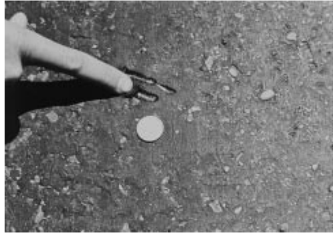
FIG. X1.5 Medium-Severity Bleeding
