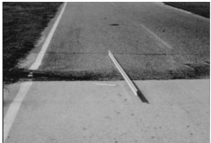
FIG. X1.46 High-Severity Shoving
