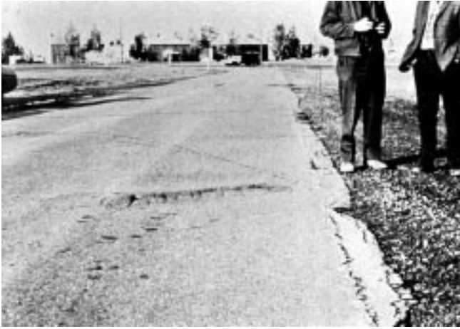
FIG. X1.11 Medium-Severity Bumps and Sags
