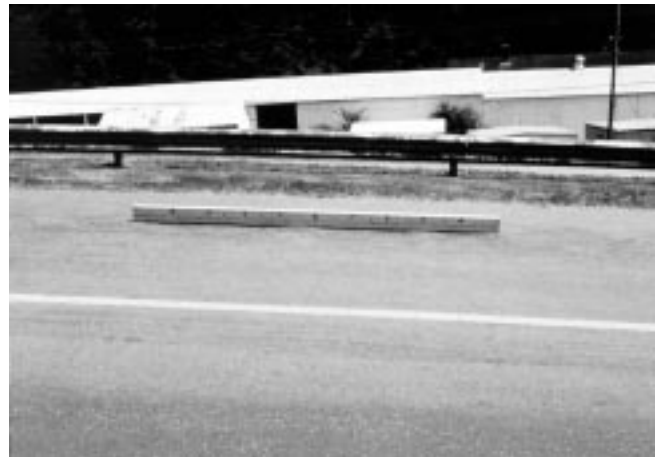
FIG. X1.14 Medium-Severity Corrugation
